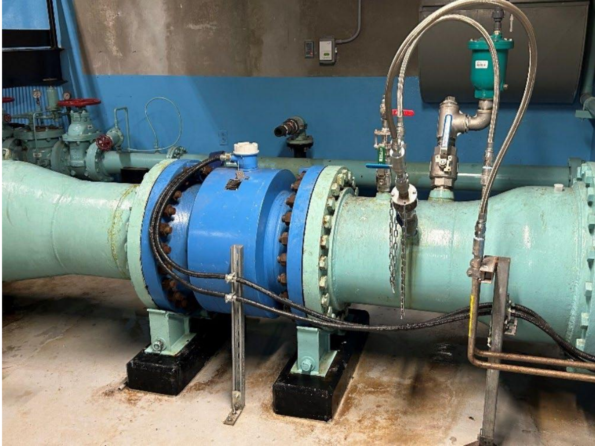
Figure 8: Completed modifications to the sodium hydroxide injection system on the west treated water discharge header.
