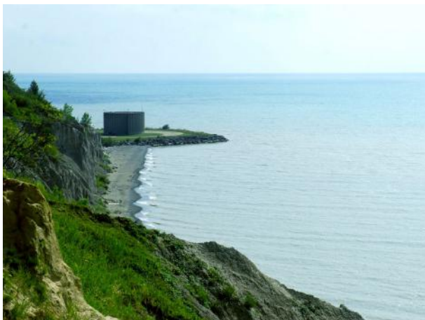
Figure 1: Low Lift Pumping Station located on Lake Erie
