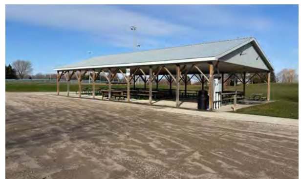
Tennis and basketball court (above), baseball diamond and supporting infrastructure (centre), pavilion and parking area (below).
