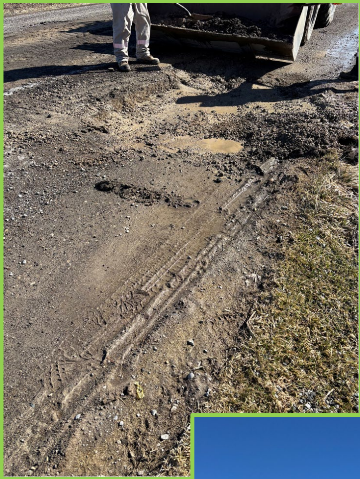
Temporary repairs completed along McBain Line.
