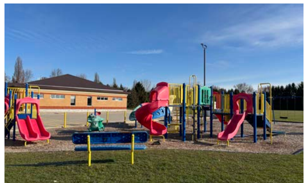
Keystone Complex and basketball court (above), fairground infrastructure and pavilion (centre), playground (below).
