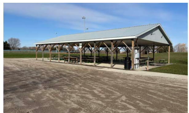
Tennis and basketball court (above), baseball diamond and supporting infrastructure (centre), pavilion and parking area (below).
