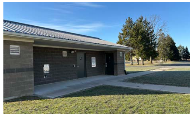
Existing path to Keystone Complex (above), pavilion and park facility (centre), washroom facility (below).
